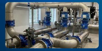
**RAINWATER DISINFECTION, IRELAND** Disinfected rainwater used for cooling of AHU's.
