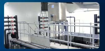
RAS\* FACILITY IN VERMONT, USA Large closed vessel UV systems for RAS\* facility.
